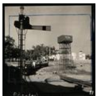
Khel Gaon Station at Bal Bhavan. (Khelgaon5_06 Dec 1959)
