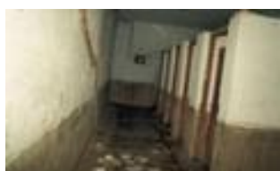
Washrooms at Anglo Sanskrit Victoria Jubilee Sr. Sc. School (LNPIII_SC031)
