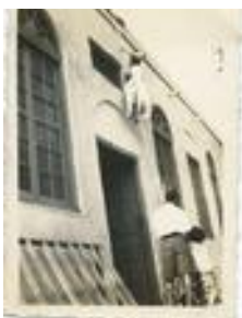
Evacuating by knotted rope-ladder. (LNP-B-025vii)
